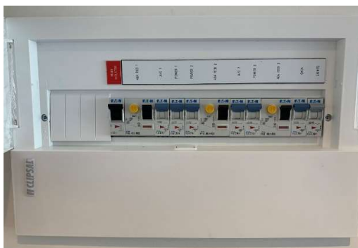
Typical apartment switchboard with all circuit breakers turned on
