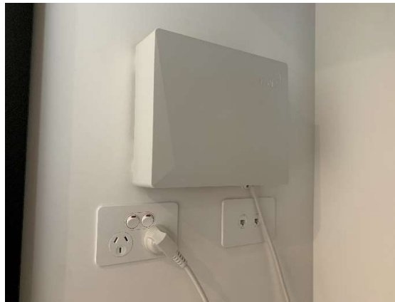
Typical NBN Box installation inside an apartment robe with robe hanging rail cut back 200mm for appropriate ventilation.
